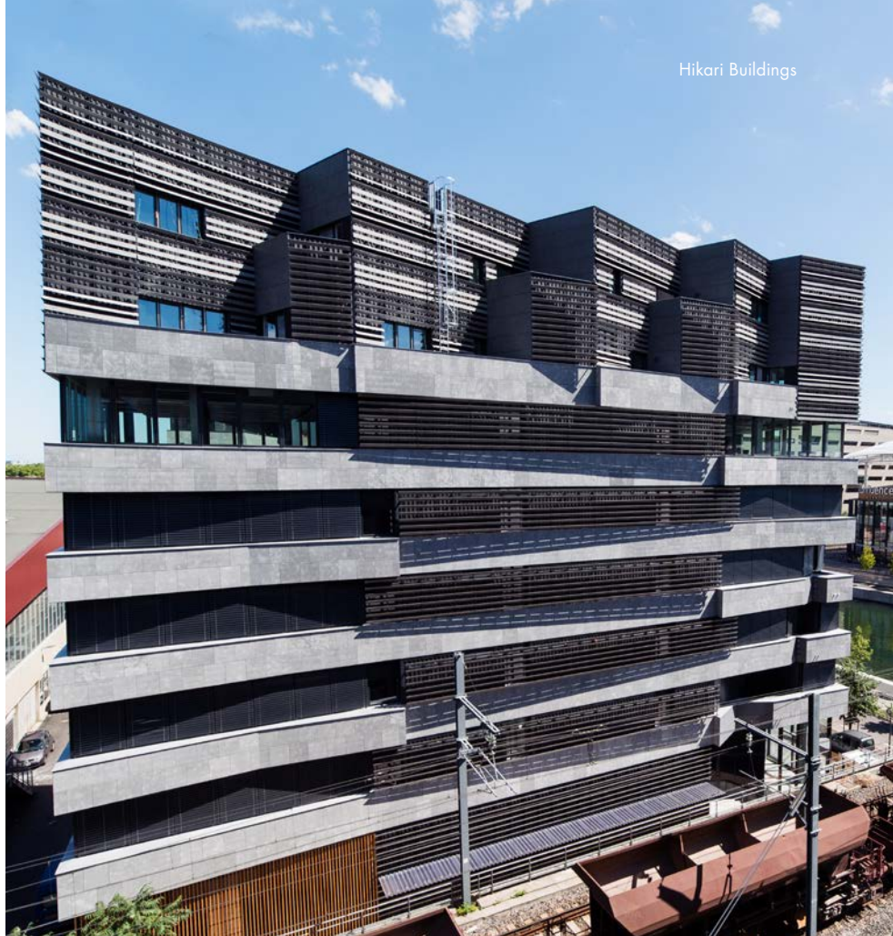
Trespa® panels were used on the top of the Nishi building
